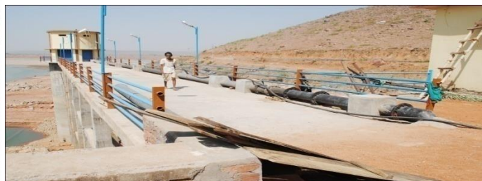
Rajghat Water Supply
